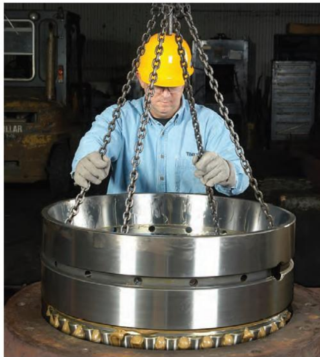
Fig. 36 Install the bottom double cone and double cup into the chock
